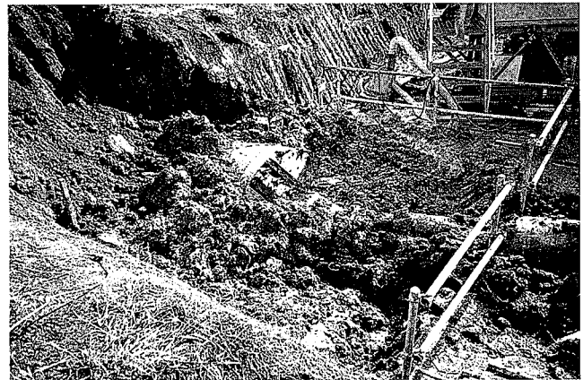
Photo 3 Arrival of dedicated cutting head at exit side
