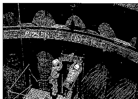
Photo 1 Installation of automatic multiple-stud welding machine to steel pipe sheet pile. Steel pipe sheet pile foundation in Takaishi section of Hanshin Bay Expressway (Owner: Hanshin Expressway Public Corporation)
