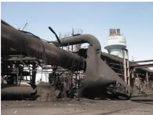
Coke gas pipe damaged by the quake
