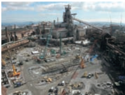
New No.2 blast furnace, undergoing foundation works (front), and No.1 blast furnace, which began operation in 2009 (rear)
