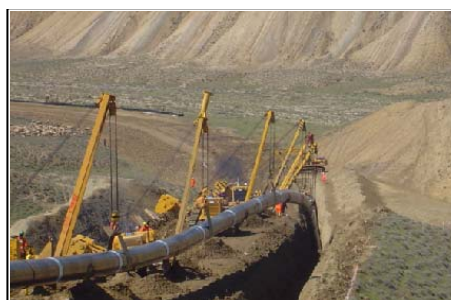
Construction scene of pipeline
