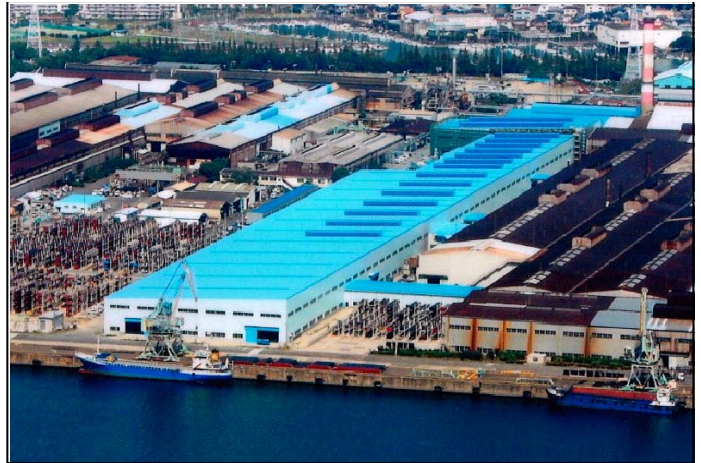
New Finishing Line Facility of the Small-size Seamless Pipe & Tube Plant at Wakayama Steel Works (located at Kainan City)
