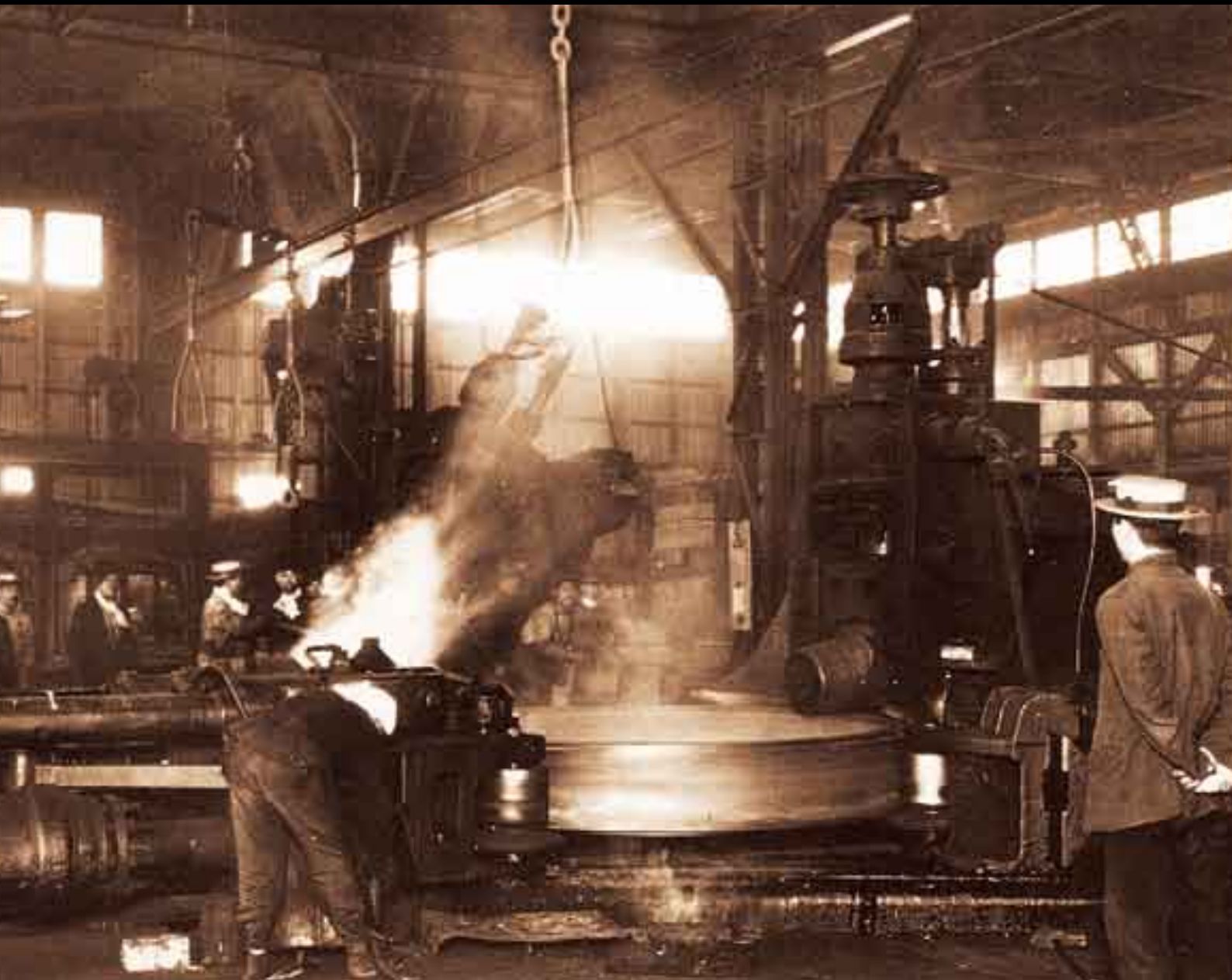
Railway wheel (outer wheel) rolling mill at Sumitomo Steel Foundry
