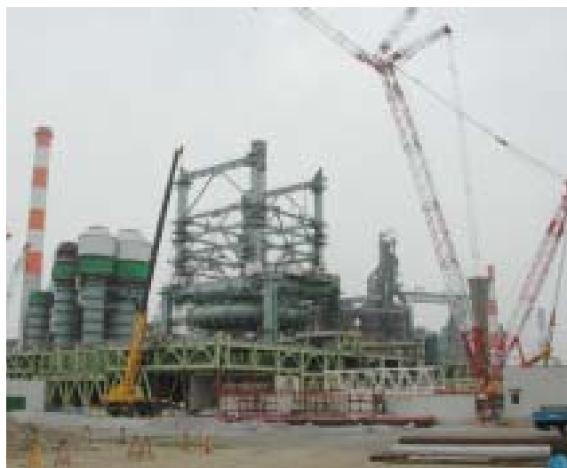
The new blast furnace under construction
