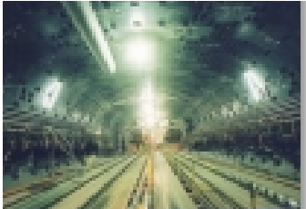
Assembling composite segments
