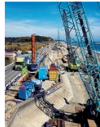
Status of construction along the Kochi coastal area
