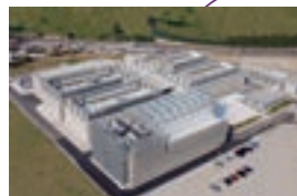
The “Kitakyushu Data Center”
