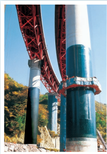
An example of the use of “Towsheet™,” a repairs and strengthening material (used as a strengthening material for a concrete structure)
