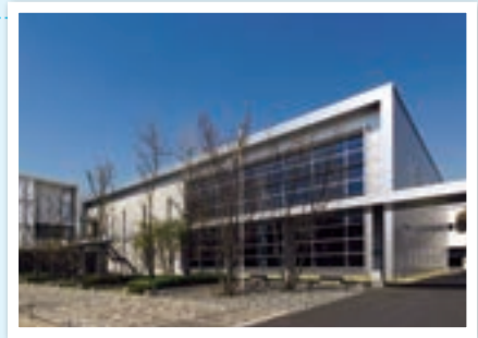
Experimental facility at the Technical Research Institute of OBAYASHI CORPORATION adopting 1,000-N grade steel
