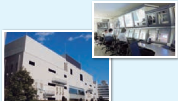
Next-generation No. 5 data center (operations room shown on right)
