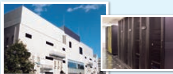
Next-generation No. 5 data center
