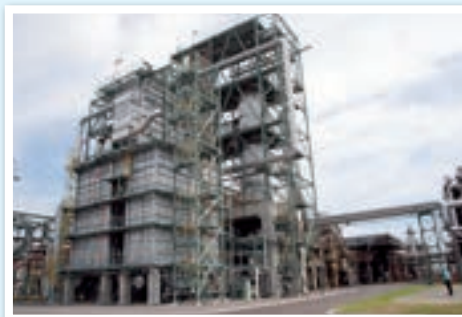
No. 2 styrene monomer manufacturing facility at the Oita Works
