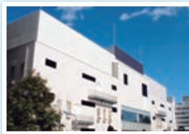
Completed number 5 data center
