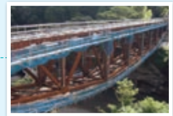
Shinmiyagawabashi bridge during construction
