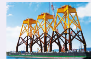
Jacket-type foundation to support offshore wind turbines
