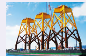
Jacket-type foundation to support offshore wind turbines
