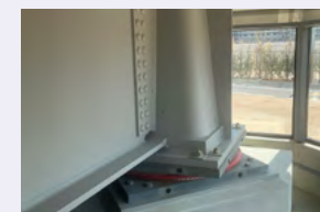
Steel-made seismic isolation devices utilizing the pendulum principle: NS-SSB™
