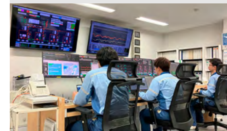
We design and construct optimal energy facilities on the premises of customers, providing comprehensive services, including O&M (operation and maintenance)
