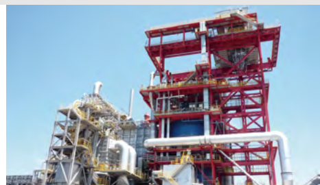
Coke dry quenching equipment (CDQ) recovers thermal energy from coke and contributes to reducing CO 2 emissions from steelworks
