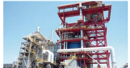
Coke dry quenching equipment (CDQ) recovers thermal energy from coke and contributes to reducing CO 2 emissions from steelworks
