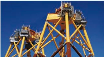
Jacket type foundation for Ishikari Bay offshore wind power plant Steel structure engineering supporting carbon neutrality
