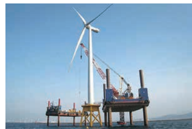
Jacketed offshore wind power generation facility under construction in Ishikari Bay, Hokkaido Photo shows demonstration facility off coast of Kitakyushu City
