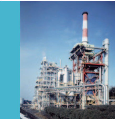
Coke dry quenching (CDQ) facilities
