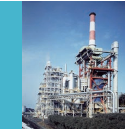
Coke dry quenching (CDQ) facilities
