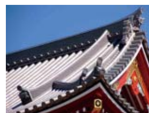
An onigawara demon tile made of Super-PureFlex and standard roof tiles on the Hozomon Gate of Sensoji Temple
