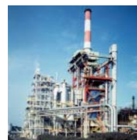
A coke dry quenching facility
