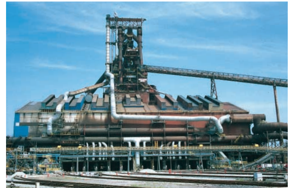
After a relining project, the No.4 Blast Furnace at Kimitsu Works is now the largest in the world by volume. The resulting increase in pig-iron production capacity will lower costs by reducing the amount of scrap purchased.
