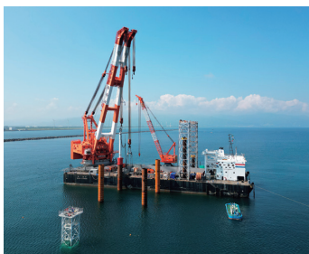
Steel pipe piles for fixing the foundation to the seabed
