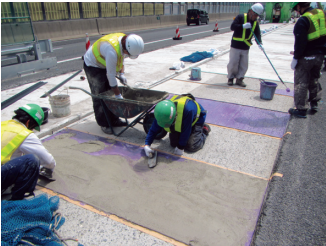
Used the CFRP “Strand Sheet™” JCM burying method that realized dramatic reduction in construction period for reinforcing highway floor panels.
