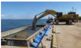
Construction using a soil modifier made from steelmaking slag
