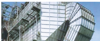
Dust generated in the burning process is collected by two types of dust collectors (electric or with bag filter), depending on the characteristics of the dust (i.e., particle size distribution, emission gas concentration.)
