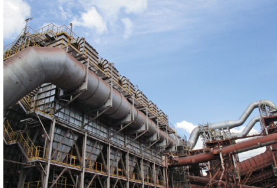
A newly-installed dust collector at the Nagoya Works
