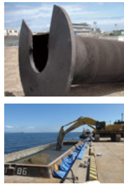
Installation of NS ECO-PILE™ and calcia modified material
