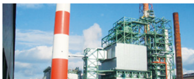
The dry desulfurization and denitrification methods, using active coke, enables SOx and NOx in emission gas to be eliminated.
