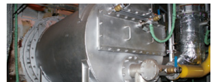
Burners featuring reduced levels of NOx generation and outstanding fuel savings have been installed.
