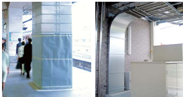
Pillar modified for earthquake-resistance inside a station
