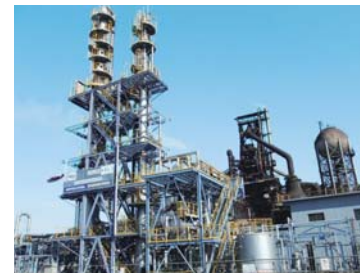
CAT30 (CO 2 absorption and separation tower)
