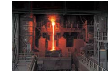
電気炉 (和歌山) Electric arc furnace (Wakayama Works)
