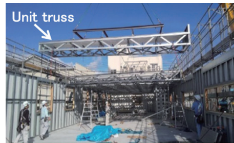
写真7 平家事務所の建方 Scene of 1-story steel framed office construction
