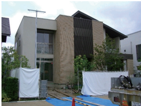
図10 開発工法を適用して不同沈下修正を行った戸建住宅 Fig.10 The house corrected by the developed method with expansive steel tubes.
