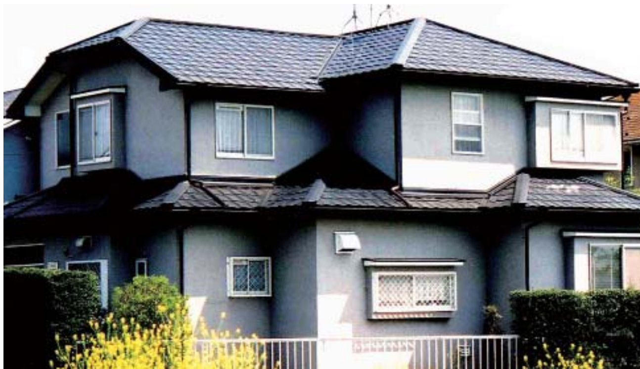
図15 開発材の住宅屋根への使用例(日新総合建材(株)製タイトルーフ) Fig.15 Application of the developed product for roofs of housing.
