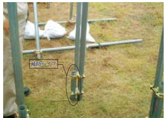
図12 補助パイプによる補強 Fig.12 Column reinforced by additional pipe.
