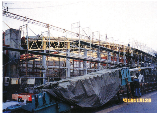
図18 富山県福岡町多目的広場新築工事 Fig.18 The multi-purpose open space building construction in Fukuoka-cho Toyama.
