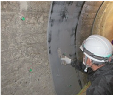
Photo 5 Adhesion work of CFSS
