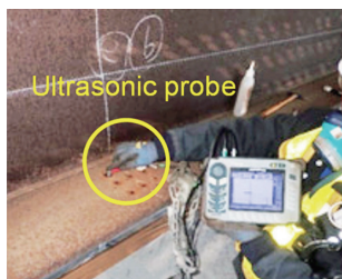
Fig. 2 On-site thickness measurement of steel plate by ultrasonic equipment
