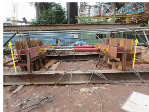
Fig. 6 Sheet pile walls after lateral loading test (Left: U-type, Right: HAT-type)
