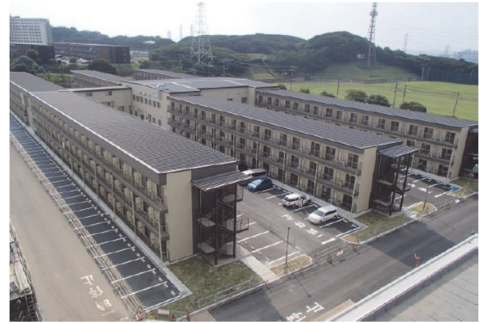
Photo 6 3-story steel framed dormitory (Source: Nippon Steel Texeng Co., Ltd.)
