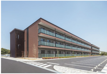
(a) 3-story steel framed house
