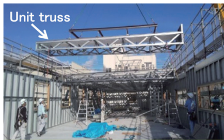
Photo 7 Scene of 1-story steel framed office construction
