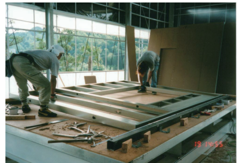
Photo 2 Scene of structural panel production in factory
