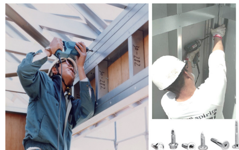
Photo 3 Jointing method for structural panel with self-drilling screw
