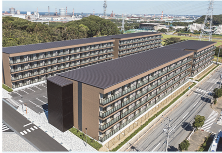
(b) 4-story steel framed house
