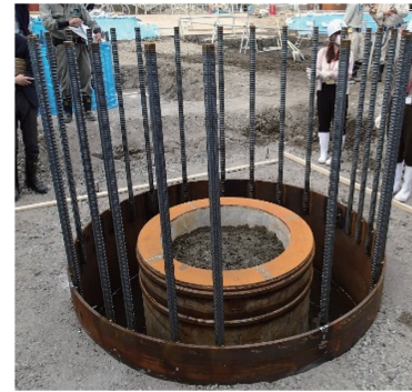
Photo 7 Setting of enlarged outer steel tube
