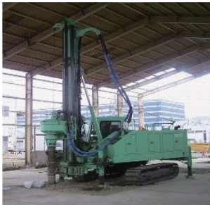
Photo 3 Small pile rotary machine 6)
