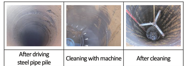
Photo 6 Before and after cleaning inside steel pipe pile
