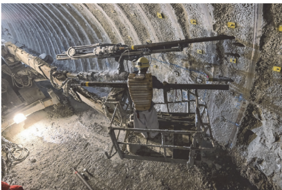
Fig. 5 Picture of AGF method with high-tension pipe 2)
