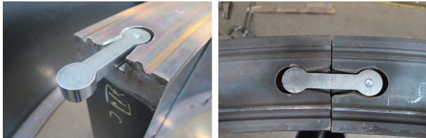
(a) "Dumbbell" joint (M) (b) "Dumbbell" joint (after fitting)
