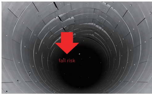
Fig. 2 Predicted damage of tunnel by earthquake
