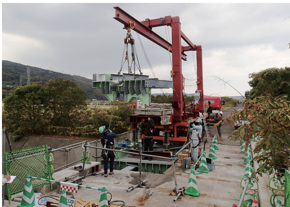
Fig. 11 Midorikawa bridge under deck replacement work
