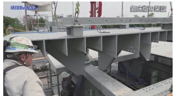
Fig. 3 Panel erection in mock-up test
