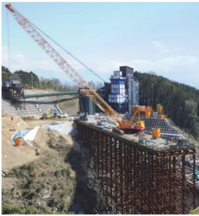
(a) Example using H-shaped steel
