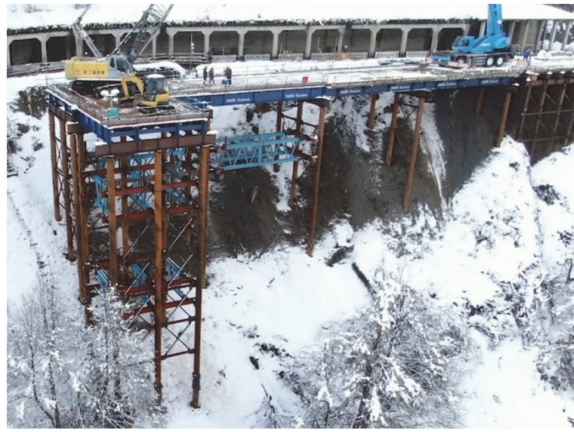
(b) Example using steel pipe piles
