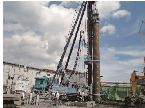
Photo 1 Inner-excavation steel piling
