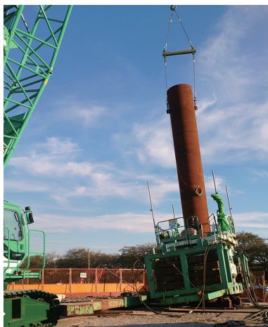
Photo 2 Batter-piling
