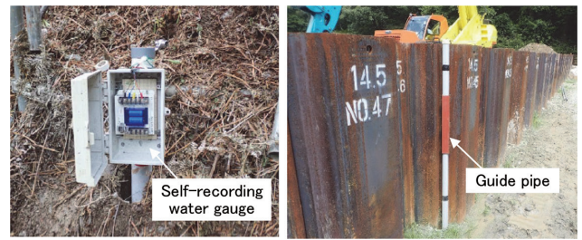
Fig. 4 State of on-site observation
