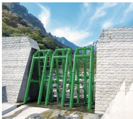
Fig. 4 Steel slit dam (AB-type)
