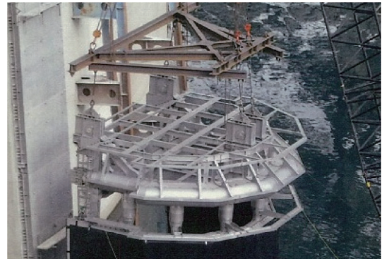
Fig. 2 Application examples of NSSC 2120 for dam facilities 4)
