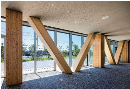
Fig. 9 Application of timber-steel hybrid fire-resistant column
