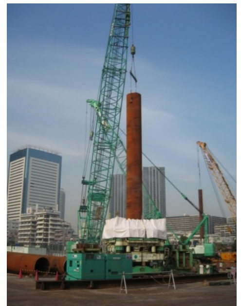
Photo 4: Deep-piling work for a high-rise condominium on soft ground
