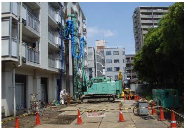
Photo 3: Piling work in a small space for earthquake-resistance reinforcement of a condominium
