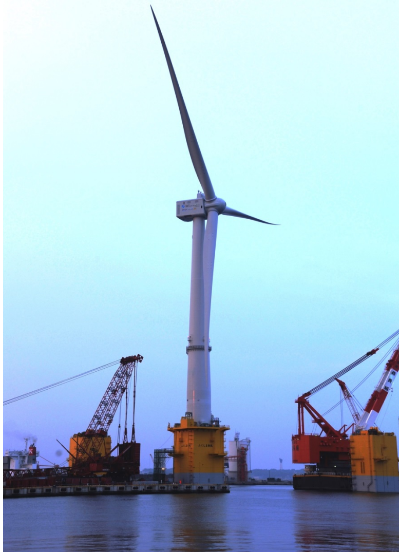
7MW Oil Pressure Drive-Type Floating Wind Turbine “Fukushima Shimpuu”
