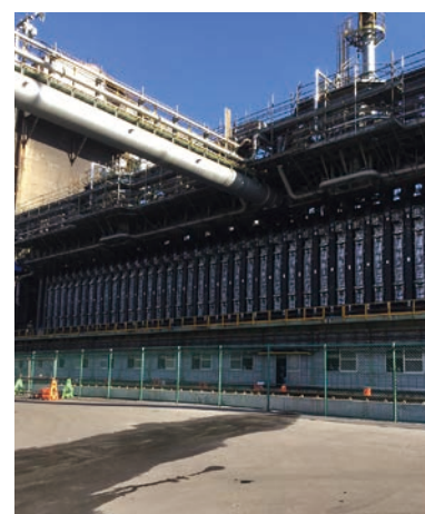
Muroran Works No. 5 coke oven (CO) refurbishment
