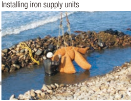
Installing iron supply units By mixing with humus, the iron eluted from steel slag is prone to be absorbed by plants without becoming oxidized.
